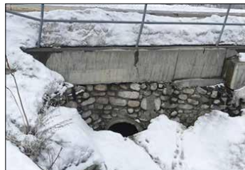
This culvert near the intersection of Seventh Street and Paradise Hill Road would be replaced with a larger one as part of the part of Brewster's proposed flood control measures.
